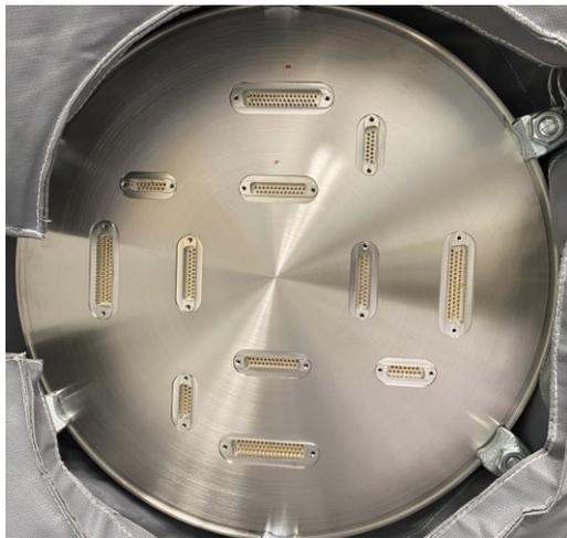
Figure 10.5 A DN320 Electrical flange with Sub-D connectors
